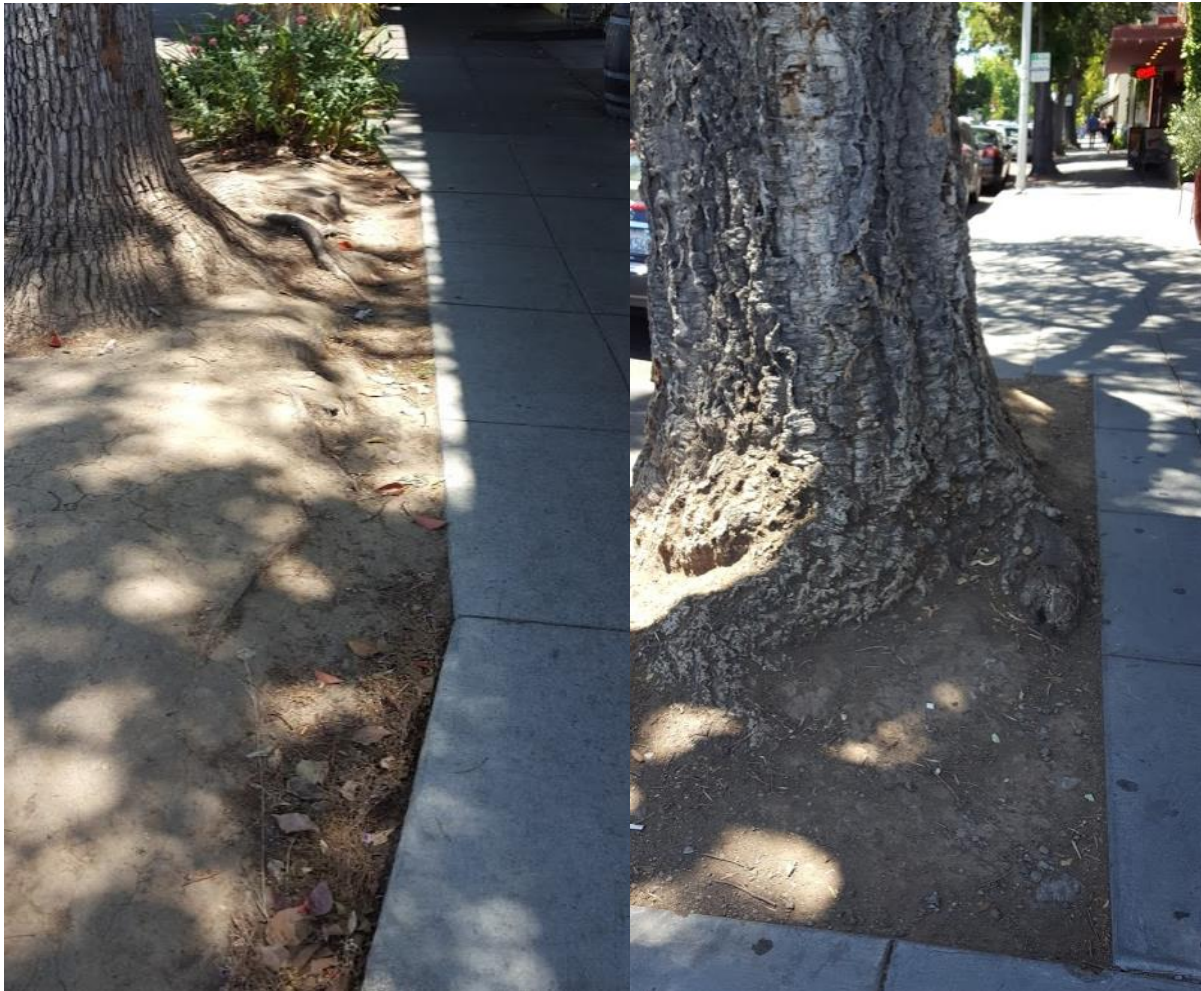
Figure 5. Camphor (Cinnamomum camphora) (left) and cork oak (Quercus suber) (right) have expanded and outgrown their narrow and small planting areas in downtown areas. Remedial treatments (sidewalk width reduction and removal) have been employed so far (Palo Alto).
