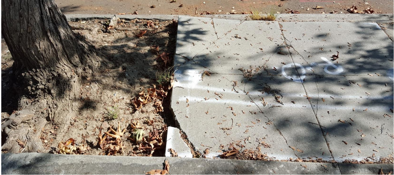
Figure 8. Example of Sidewalk Repair Program marking cracked/lifted concrete adjacent to a street tree to be removed and not replaced in order to increase the planter length (Palo Alto).
