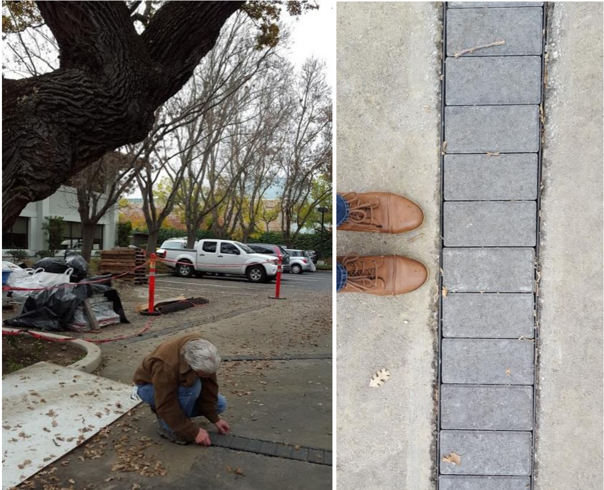
Figure 35. Root path installation radiating out into parking lot to improve the root zone of a high-value tree (Palo Alto).
