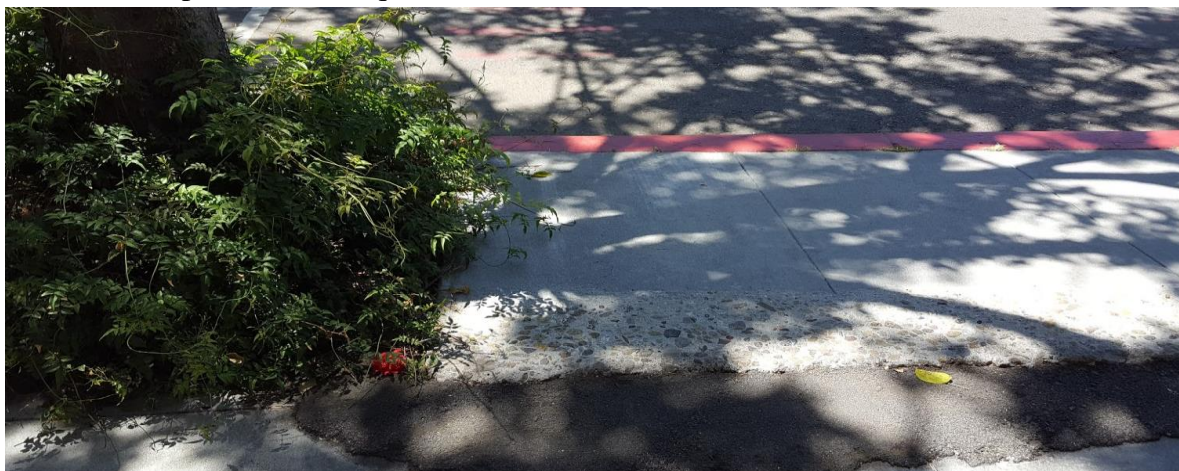
Figure 24. Example of asphalt shim used next to street tree (Palo Alto).
