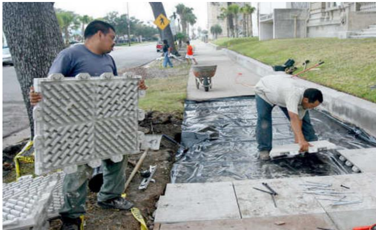
Figure 31. Photo of Terrewalks® installation in Galveston, Texas.
