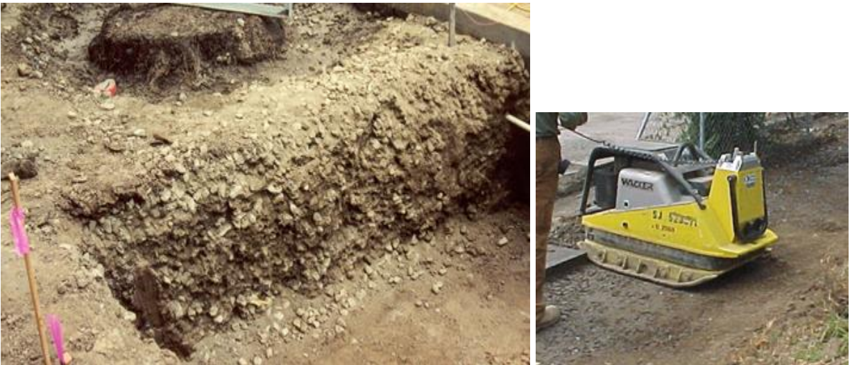
Figure 37. Engineered Soil Mix in trench during installation (left) and equipment used to compact the ESM for engineering standards (right).
