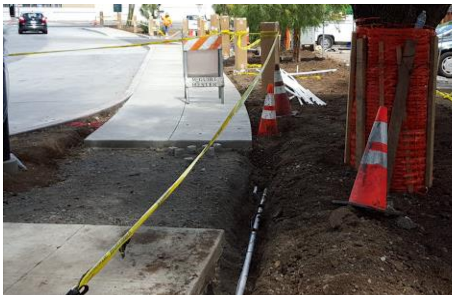
Figure 28. Site preparation prior to rubber sidewalks (Terrecon, Inc) installation adjacent to existing trees for a new walking path (University Circle, Palo Alto 2016).
