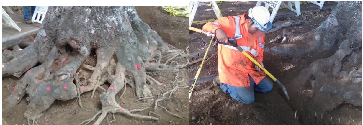
Figure 6. City of Palo Alto uses their air spade to employ minimal impacts during tree root excavation prior to determining allowable root pruning.
